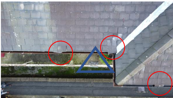
Evidence of Slate slippage on eaves course . Ageing of slate leading to higher moisture content indicated by darker areas & potentially leading to the softening of Slate.
