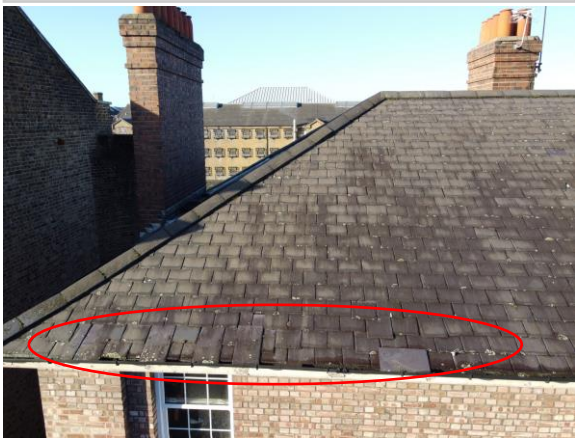
Evidence of Slate slippage on eaves course . Ageing of slate leading to higher moisture content indicated by darker areas & potentially leading to the softening of Slate.
