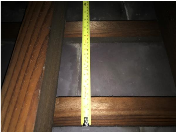
Image confirming existing batten gauge, 200mm, Slate lap, 100mm.
