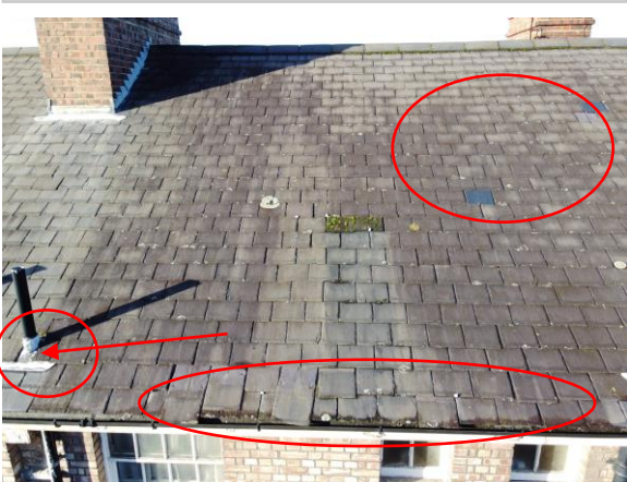
Faulty slate to Soil Vent Pipe and missing balloon. Very strong evidence to support ageing of slates and tile slippage and nail sickness. Localised remedial repairs not in keeping with fabric of roof.
