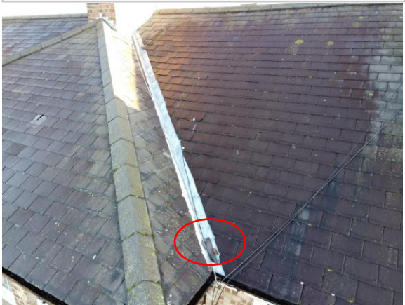
Further evidence of Slate slippage in the valley, as before described.
