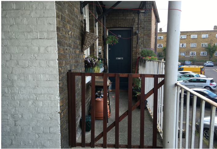
Fig 3; The external timber gate and stored items within the escape route should be removed and the escape routes kept clear at all times.
